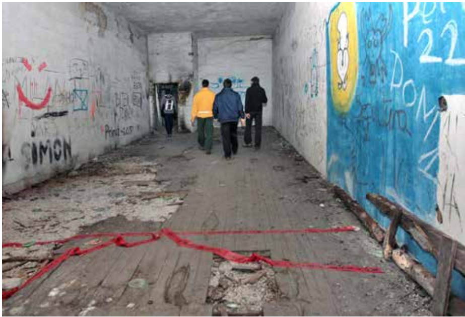
In Bunker 2 one chamber has wooden flooring. Through the opening at the end leads to steps up to a high level surface entrance that is now bricked up. Photo Žiga Ribič
